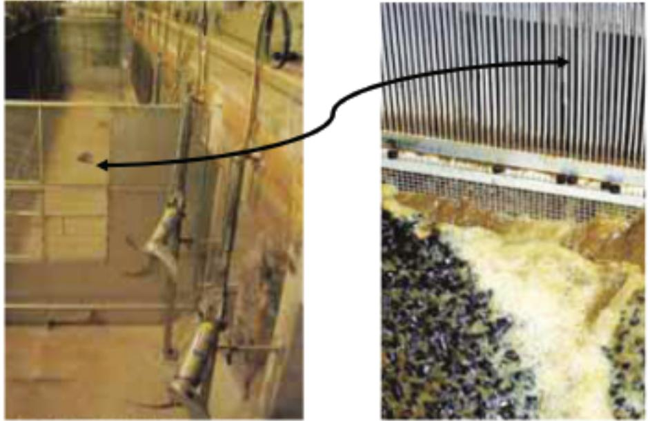
Figure 4. Flat-screen walls at each end of the aerobic IFAS zone of the Raisioplant Bardenpho process (left). Improvement to the originally designed flat-screen wall following an initial hydraulic failure that resulted in carrier loss from the Raisio plant (right).
