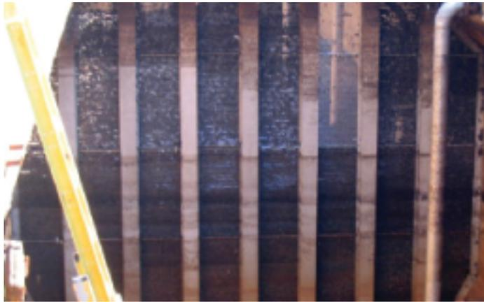
Figure 8. Plastic biofilm carrier retention flat screen with carriers lodged in screen openings
