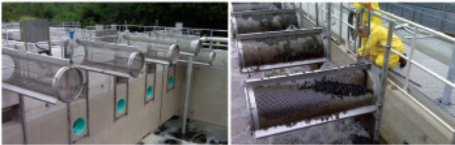
Figure 5. Plastic biofilm carrier retention screens at the Groton facility before (left) and after (right) a storm event and their structural failure
